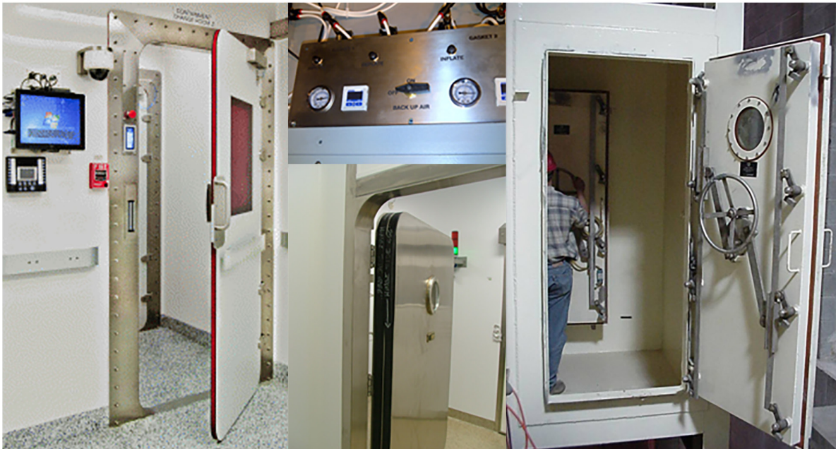
Figure 1.F. Mechanical-seal or inflatable-seal walkthrough doors. The top schematic describes how the door seal inflates to block the flow of air between rooms of a containment facility. The bottom images show examples of inflatable seal doors (left, centre) and mechanical seal doors (right). Note the red (left) and black (centre) colors of the inflatable sealing gasket.
